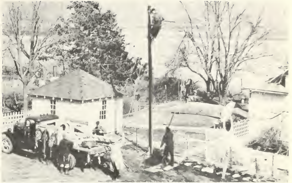
Considerable planning went into the placement of poles. If a windstorm was to topple this one, it would not strike the building. Note storm cellar behind house.
